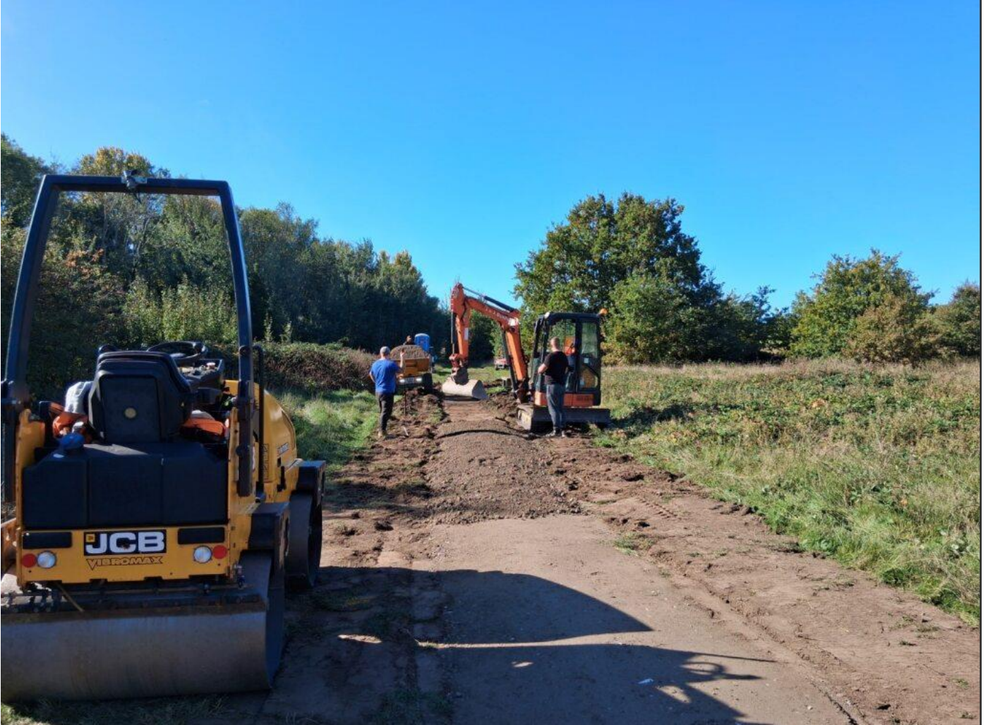
Installation of new footpath from Galpins Road to BP garage
